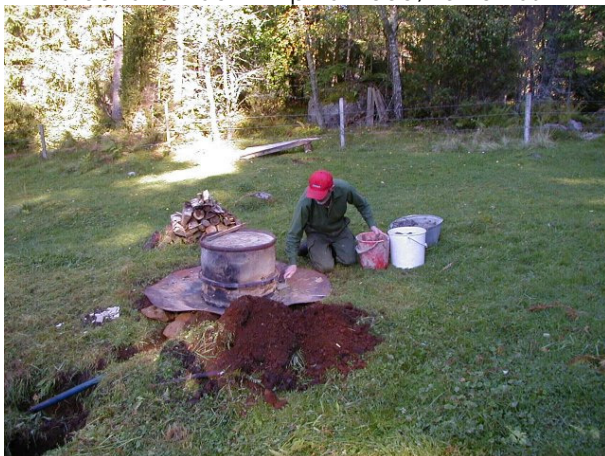
I use the clay and sand to tighten around the barrel.
